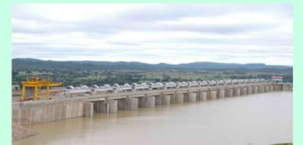
Bansagar Dam- Head Works
