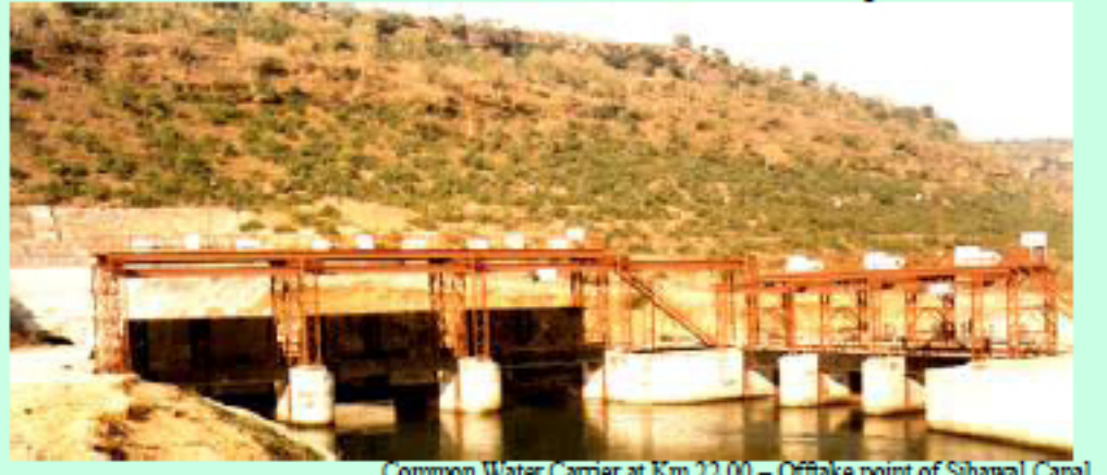
Common Water Carrier at Km 22.00 - Offtake point of Suhawal Canal
