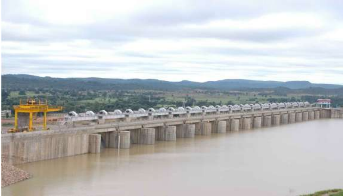
View of Bansagar Dam
